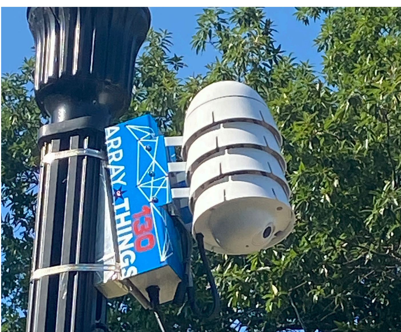
Figure 1: AoT Node installed on a light pole in front of the Computer Science building at NIU
